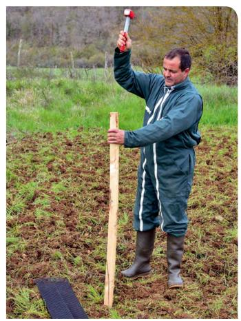
Drive the post in straight with a lump hammer or sledgehammer to a sufficient depth to keep it upright
